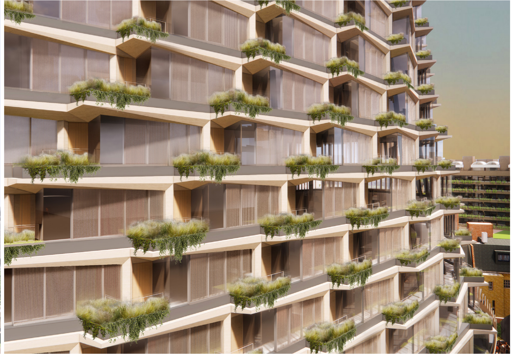
Inwards facing planted facade
