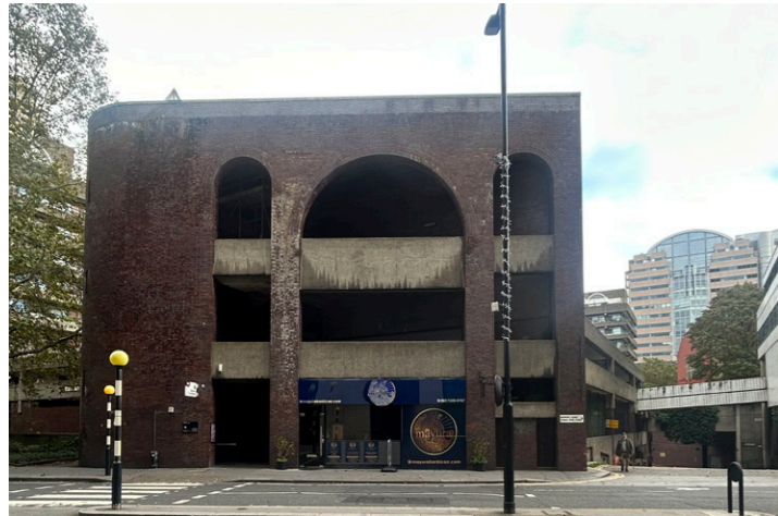
Barbican stair tower immediately North of the Site
