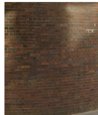
Barbican Stair Tower
