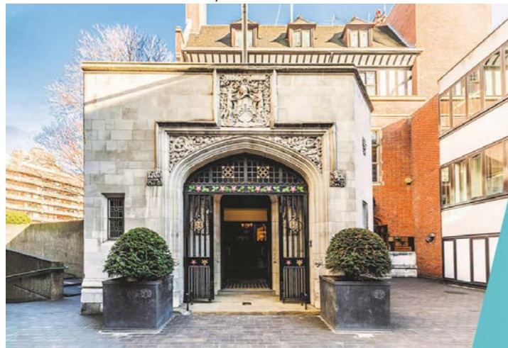
Pointed stone archway at Ironmongers' entry porch
