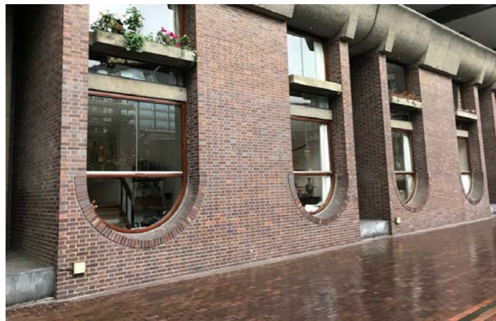
Language of brick arches within the Barbican estate (in this case, inverted)
